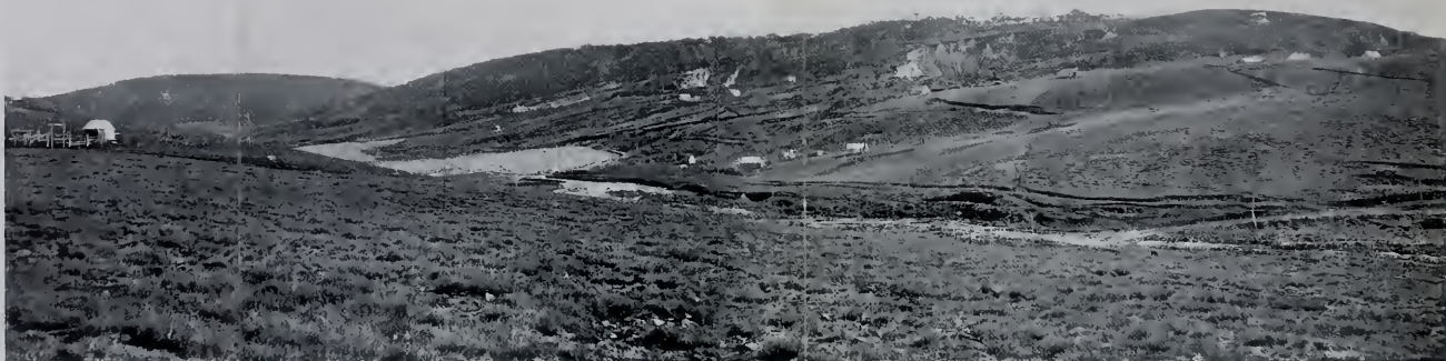
NEW CHUM HILL, SHEWING OPEN CUTS. FROM THE SOUTH.
